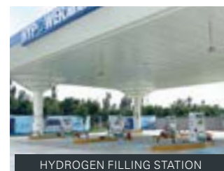
HYDROGEN FILLING STATION
